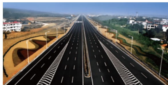
Ruili to Menglian Expressway Electromechanical Project
