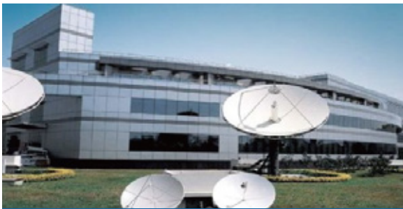
Shanghai Securities Waigaoqiao Earth Station
